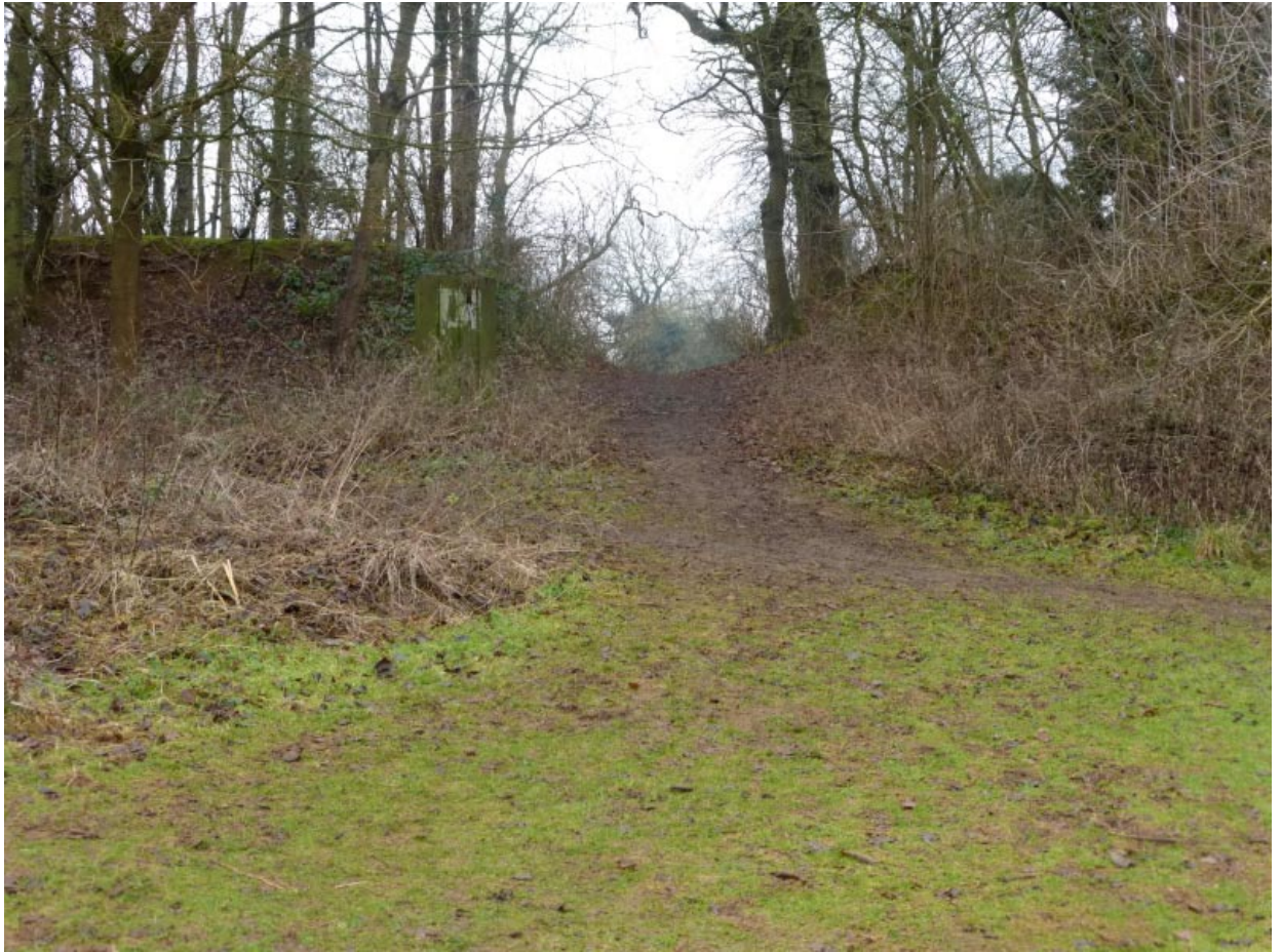
12: This illustrates the extent to which C19 open-cast quarrying has reduced the level of the ground surface both inside and outside the ditch and its banks.
