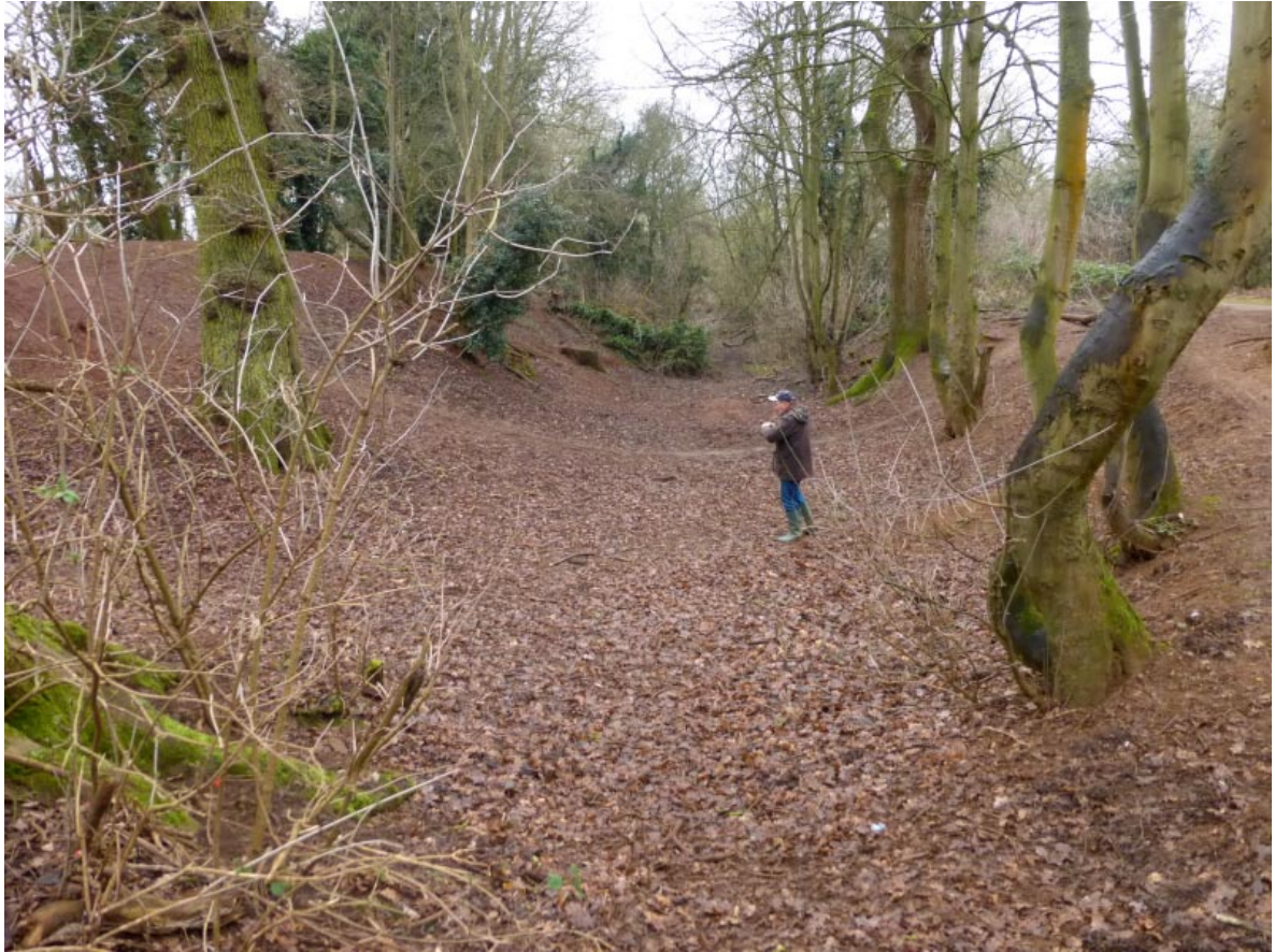
8: the ditch on the north-east side. Tree-roots are actually the only things that are keeping some parts of the ditch walls in place!
